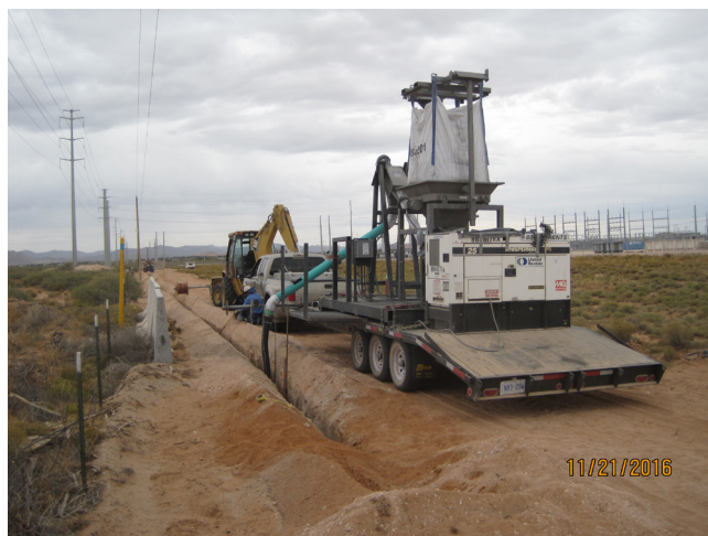
Figure 2. Compact design allows for use of 2200 lb super sacks of Conducrete for a fast and efficient placement.
