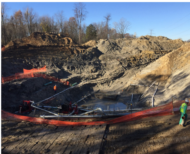
Figure 5. Large scale post-construction HDD excavation and repair.
