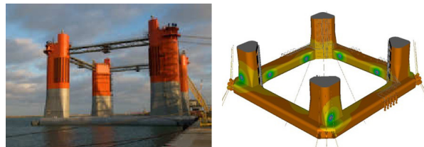
Exmar's Opti-Ex platform, unacceptable IR-free potentials after 10 years of service life with original CP design
