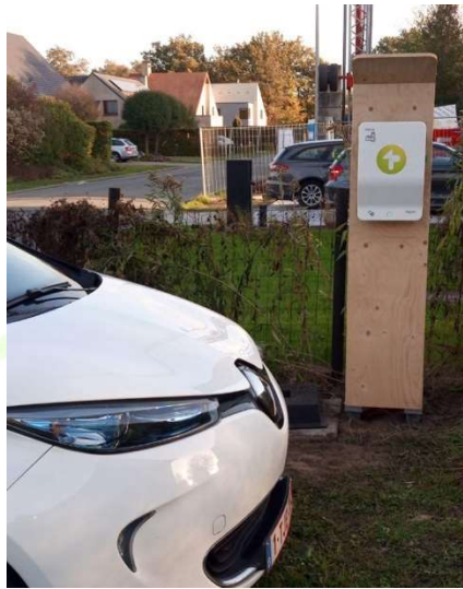
Figure 11 – EVSE installed at the Jacob's nest.
