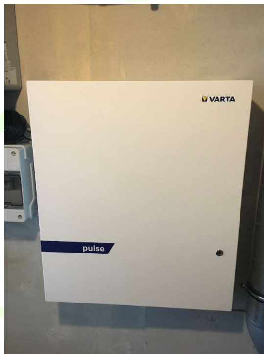
Figure 8 – Varta Pulse 6 system in DSds cohousing (location 1 of 4).
