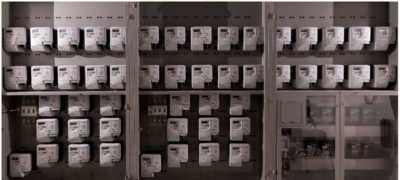
Figure 72 – SLAM installation in an apartment building in Terni.
