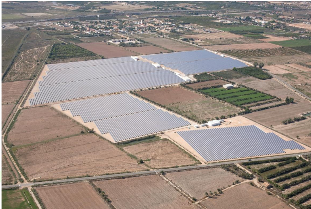
Figure 35 – Solar farm “El Realengo”
