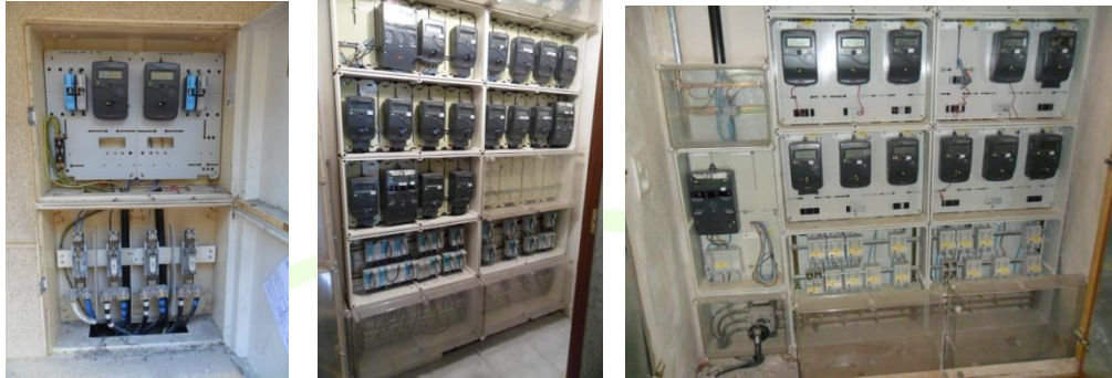
Figure 45 – Centralized meters
