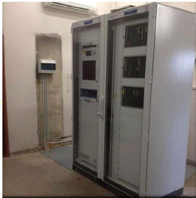
Figure 74 – EFACEC Remote Control System
