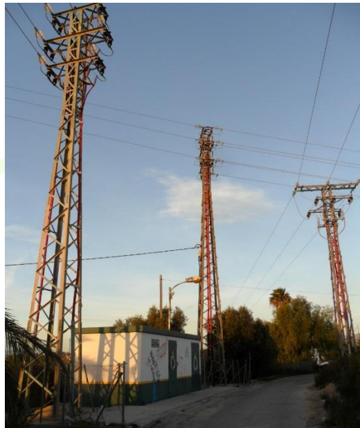
Figure 33 – Power transformer for the redistribution of energy
