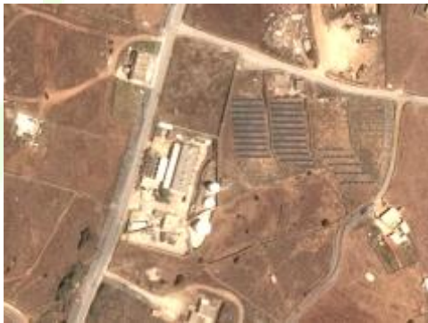
PV station Other investor 1
