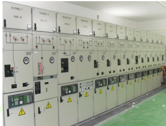
Figure 31 – 20kV protection cubicles
