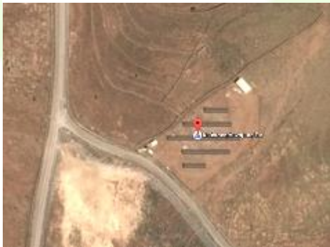
PV station Other investor 2
