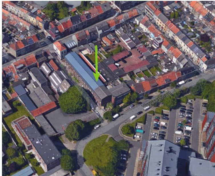
Figure 50 – Coworking site The Watt Factory – Ghent
