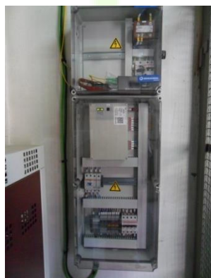
Figure 42 – PRIME concentrator installed
