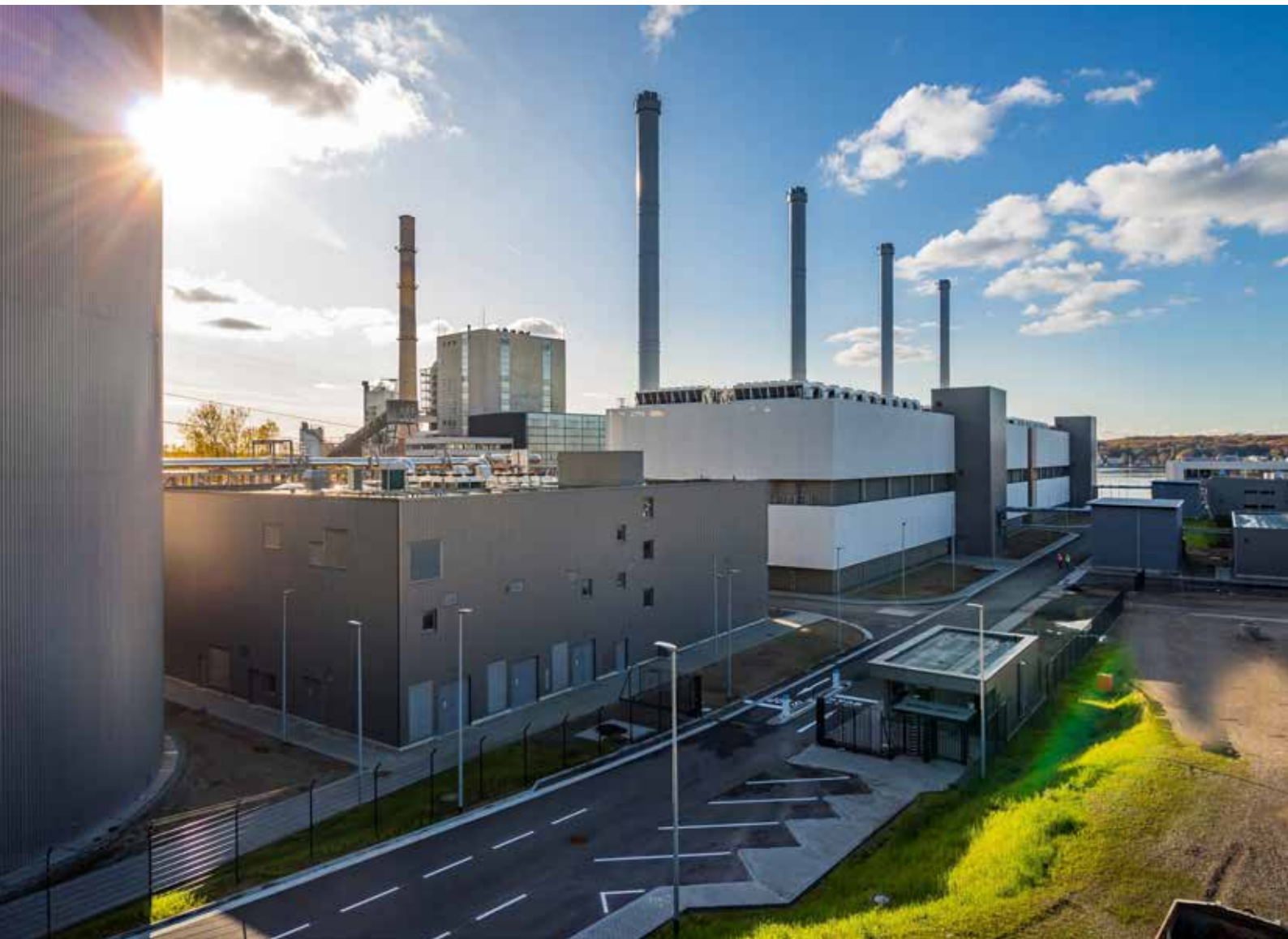
K.I.E.L. coastal power plant
